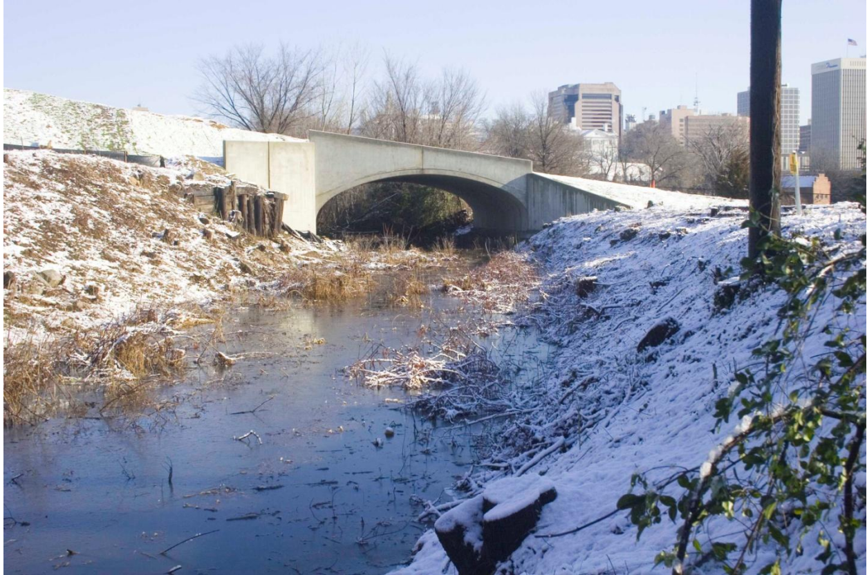
(Figure 12.) In 2012, the Richmond City Council approved the expenditure of $385,000 to protect the canal by constructing this bridge over the canal as part of the construction of the 2 nd Street Connector.
