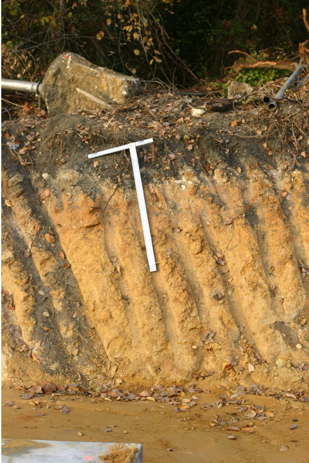
(Figure 63.) This cross section of the canal was revealed when the 2 nd Street Connector was constructed in 2012, adjacent to the site of Venture Richmond's proposed amphitheater. This cross section exposes the intact layer of the clay that was "puddled" in a process to make an impermeable water-tight canal bank. The James River and Kanawha Canal was a carefully engineered structure, designed to withstand the vicissitudes of weather and traffic, while holding back the considerable volume of water in the canal. (Source: OHHIC)
