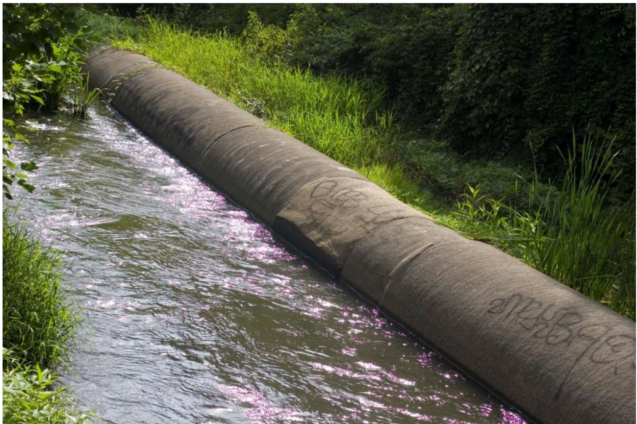
(Figure 43.) The 48 inch Korah 2 water transmission pipe installed in 1984 is shown in the bed of the James River and Kanawha Canal below Hollywood Cemetery. In order for canal boats to clear this water transmission pipe in the bed of the canal when the canal is re-watered west of Tredegar, the elevation of water in the canal must be maintained at its historical level of 83 feet above mean sea level. (Source: OHHIC)
