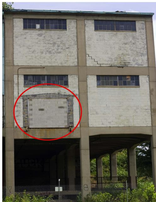
New cinder blocks are visible on the west elevation of Intermediate Terminal #3 where the elevated covered bridge connecting the building with Terminal #2 was originally located. The elevated bridge was removed when Terminal #2 was demolished in 2007.
