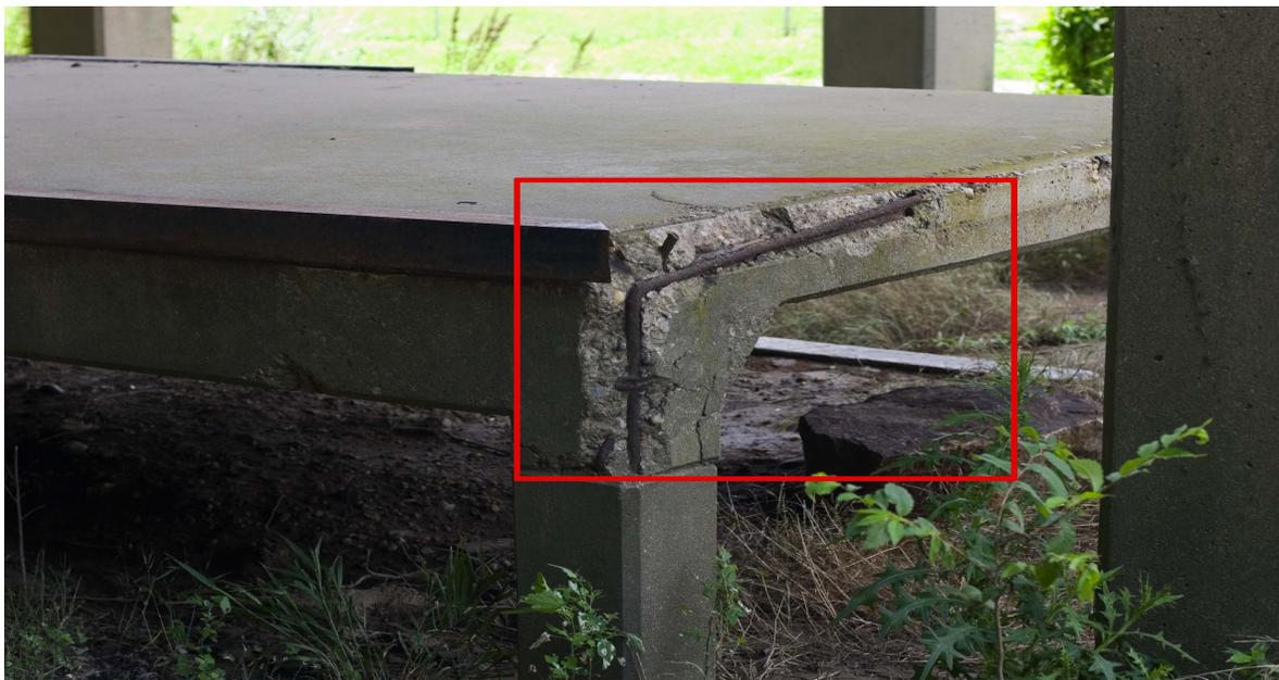
The steel reinforcing bars are visible today on several portions of Terminal #3 (cont.)
