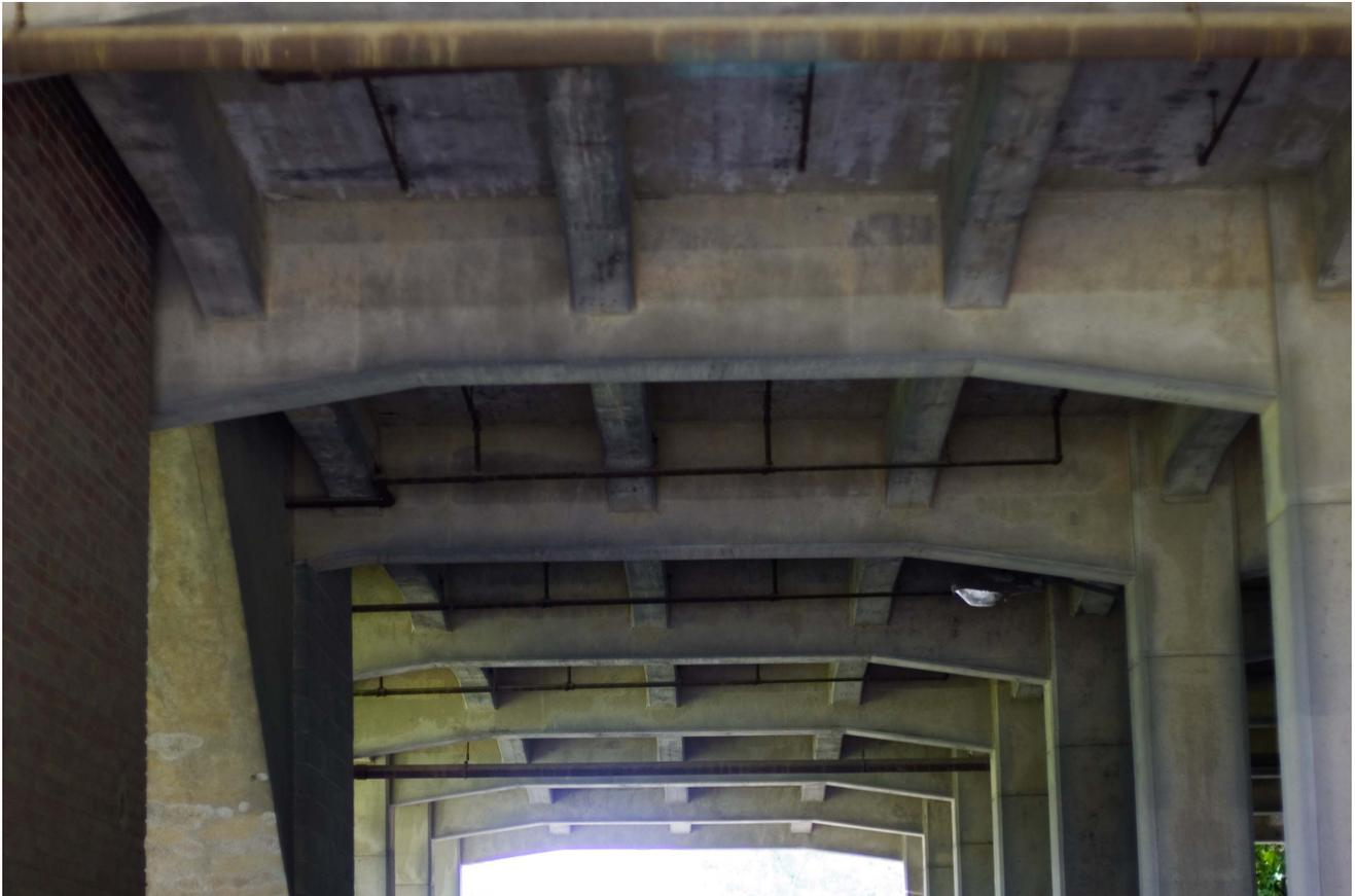
View from under Intermediate Terminal #3 shows the monumental reinforced concrete beams and piers that were designed to provide prodigious support for tons of commodities stored in the warehouse.
