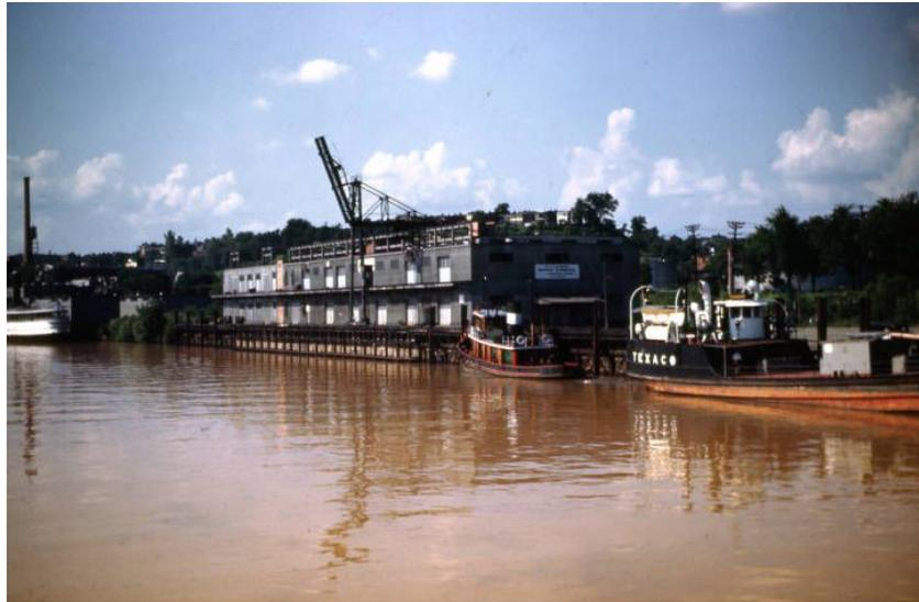
Intermediate Terminal #3 in 1944 (highlighted in detail below). Note the crane that rolled on the wharf and steel superstructure on the roof of Terminal #1. Source: VCU Archives.
